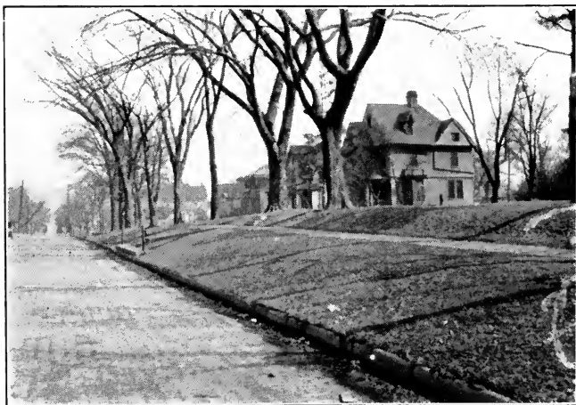
SIDEWALK AND ROADWAY AT DIFFERENT LEVELS Occasional handling in this way lessens engineering problems, saves expense in construction, and often contributes to the interesting appearance of a street.
